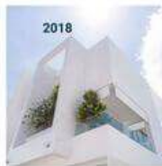
THE RESIDENCE BY ANDAMAN ASSET SOLUTION
